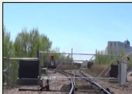
Custom Curb Notch
